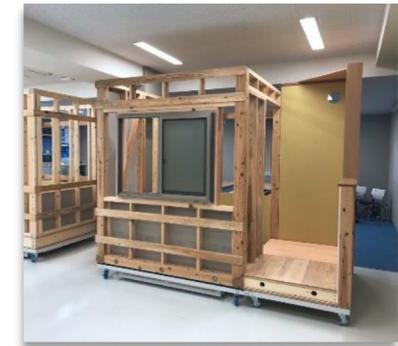
The training includes hands-on experience in product assembly and other on-site processing, as well as on-site installation checks prior to the installation of products.
